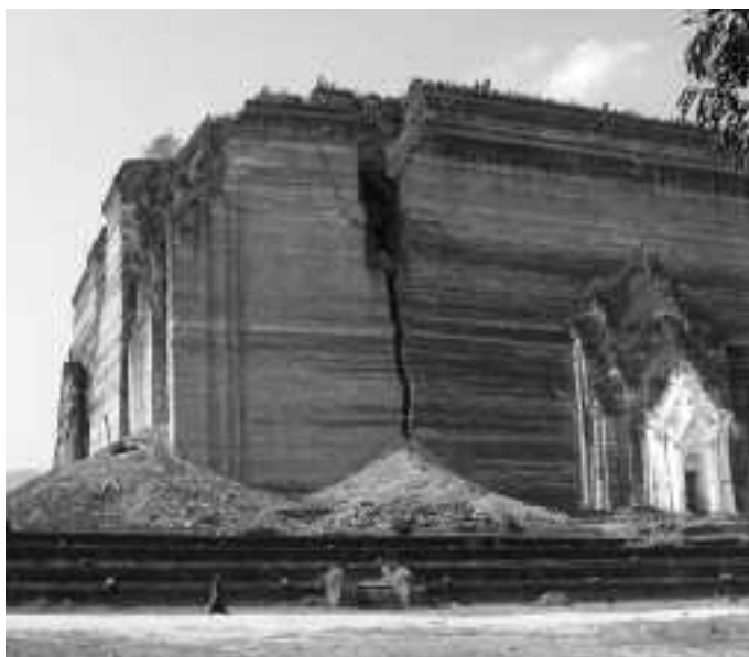
Figure 1. Construction began on the Mingun Pagoda in 1790 by the King of Burma, Bodawpaya. It was common practice to bury highly prized possessions in the pagodas. Earthquakes (in 1838) have significantly damaged the structure, but it is still a formidable building. A monk walks along the foundation in the foreground. Photograph by the author, 2006.
